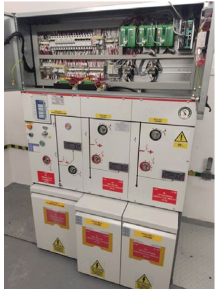
Fig.2 Interior of the T-2846 Mickiewicza Sopot secondary substation after modernization, including the information board, transformer and MV/LV switchgear, (Energa-Operator SA, 2023).
