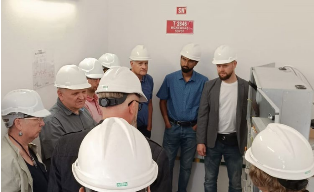
Fig. 5A, B SUSTENANCE Partners visiting the modernized T-2846 Mickiewicza Sopot secondary substation on the 1st of June 2023 (Energa-Operator, 2023).
