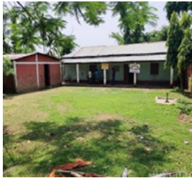
Case 2: BORAKHAI VILLAGE, which aims at delivering smart clusters based on local energy systems powered by renewables
